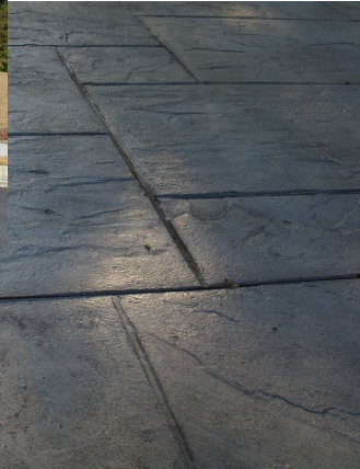
Installing a patio
